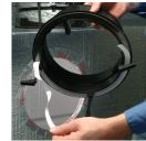
Insert Collar: Slightly push in heads of Quick Zips to fit into pre-cut hole in duct board or sheet metal trunk line. Push collar against trunk line surface. Once pressed in place the adhesive gasket will adhere to surface.
