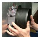
Pull Quick Zips Tight: Pull each Quick Zip tight by bracing base of palm on collar edge and pulling to lock collar in place. The Start Collar is universal and will seal tight to sheet metal, up to 2" duct board or insulated duct. If sheet metal is used, a standard zip screw can also be used to secure using the 4 predrilled holes in the Start Collar's outside flange.
